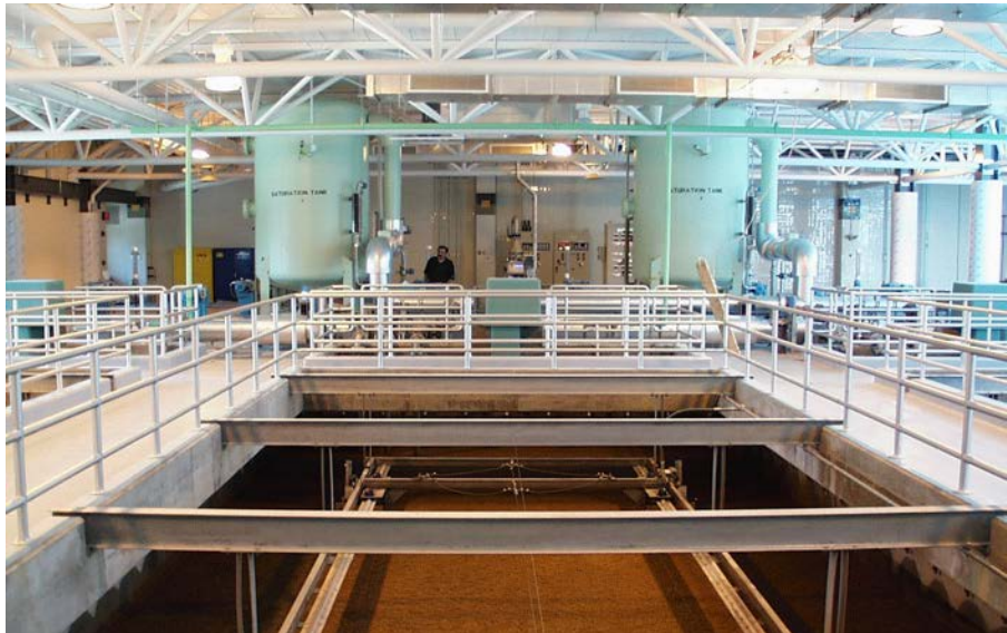
TYPICAL DAF INSTALLATION
