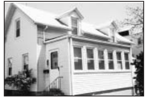
The owner-occupant of this Pine Street home would have saved over $700
