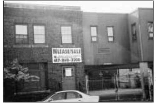
Site of the proposed development on Hampshire Street
